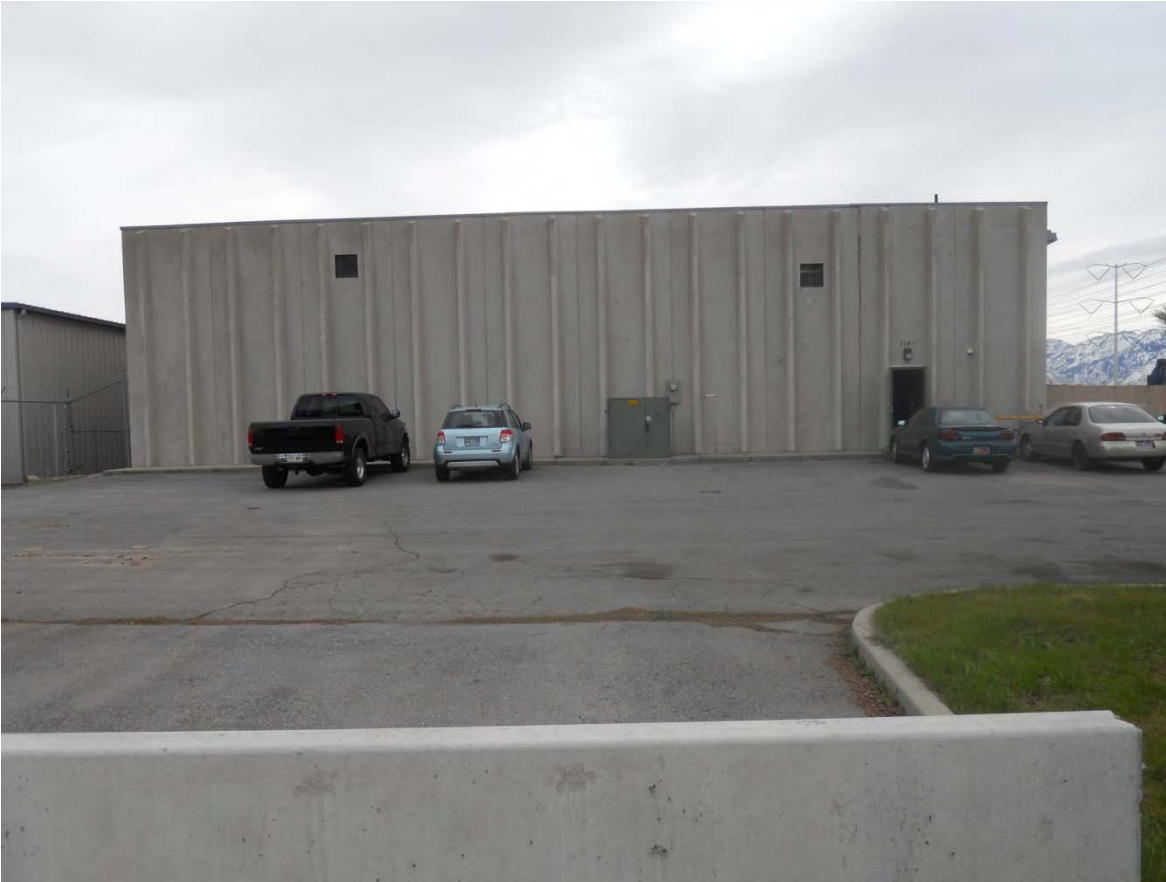
Looking at the main building which is located on the east side of 3200 West.
